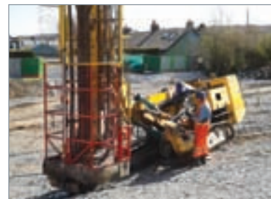
Typical rig guarding now in common use
